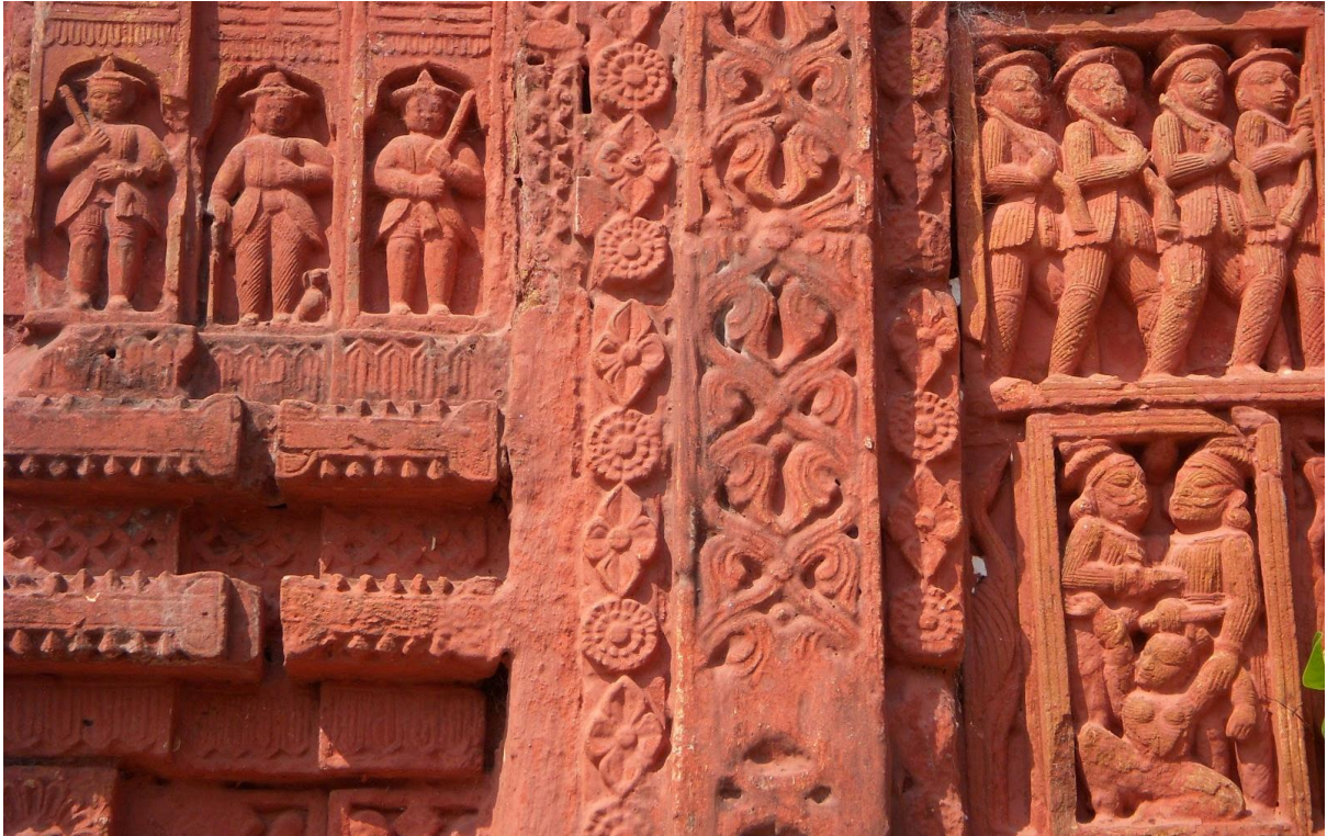
Image No 76 : Anondomoyee Temple Wall Terracotta at Sukharia, Balagarh
