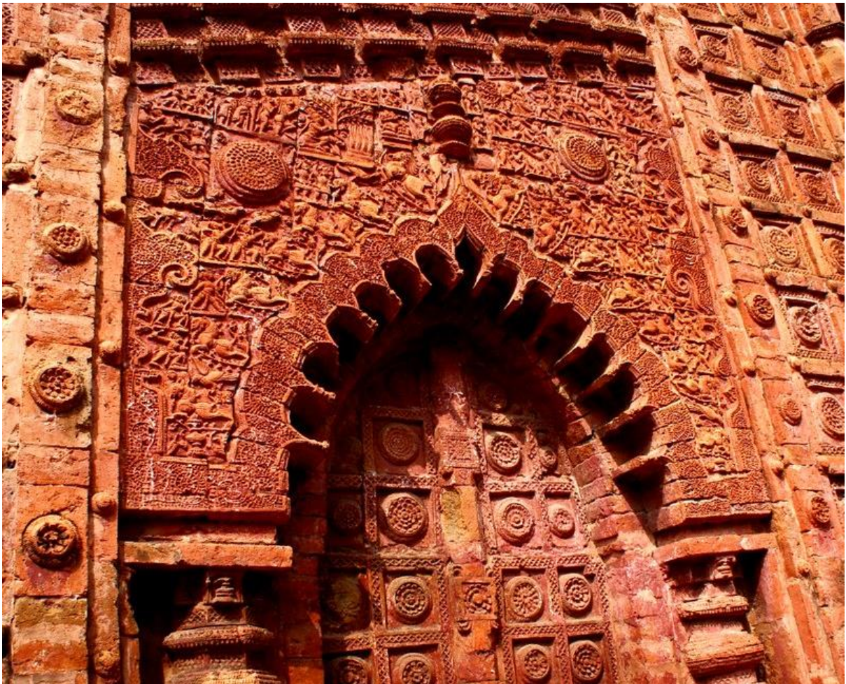
Image No 77 : Anondomoyee Temple Wall Terracotta at Sukharia, Balagarh
